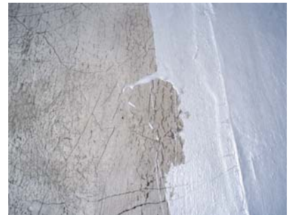
Lucas #3000 flows into cracks and gaps sealing the surface. Smoother surfaces drain water more efficiently and prevents the cracks from developing into leaks.
