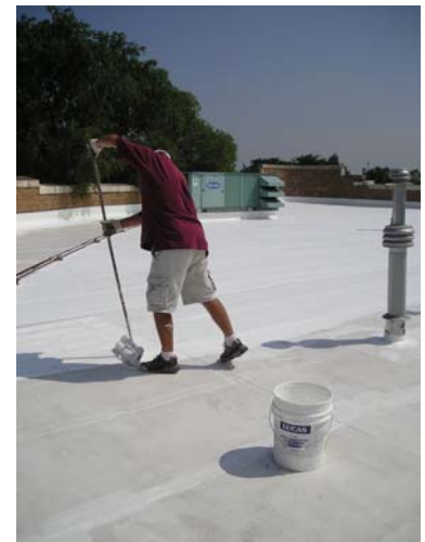
Lucas # 1000TC is applied over an initial coat of Lucas #1000MB.
